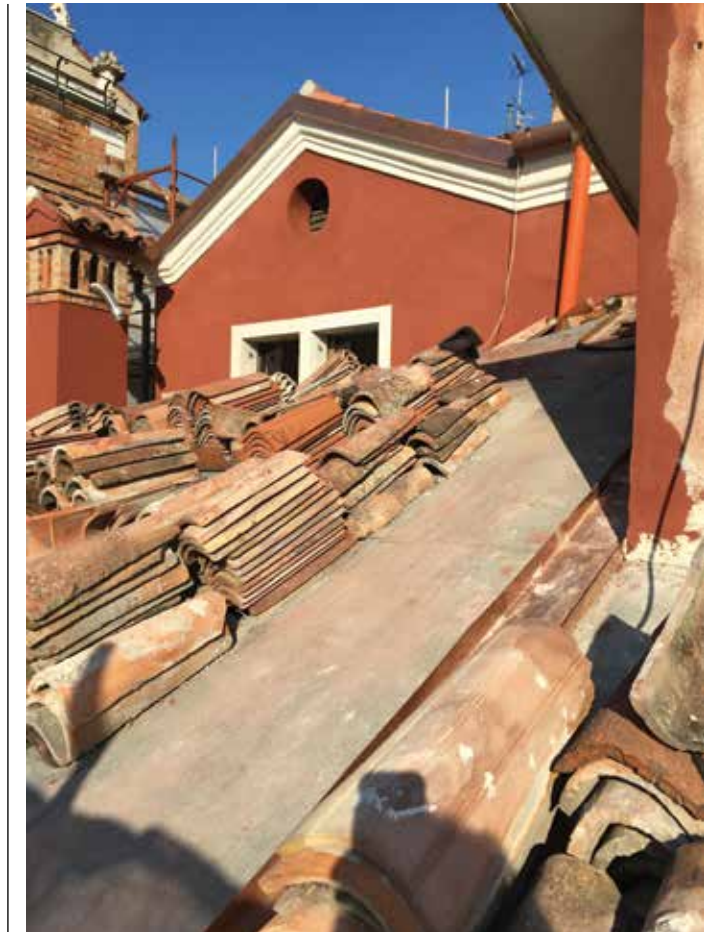
Casa Muraro during renovation. Photograph by Holger A. Klein.
