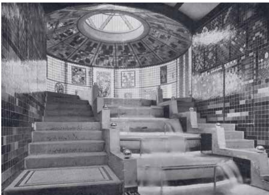
The Glass House by Bruno Taut, Cologne Werkbund Exhibition, 1914. Interior view from the lower part of the cascade room with the oculus to the exhibition hall visible at the top of the cascade. Taut's brochure credits the many artists, artisans, and companies that provided the experimental construction materials, glass prisms and brick, stained glass, metalized ceramic tiles, glass globes, and other new uses of glass and concrete documented in the installation views illustrating this essay (see page 105).
